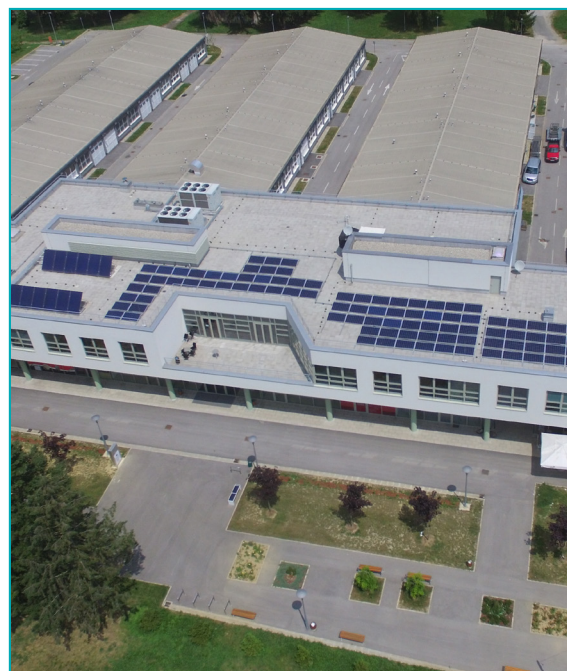
PV plant. - © Križevci
